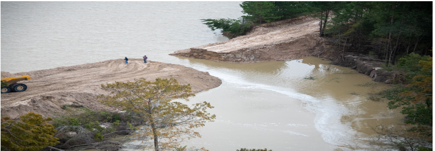
Liberty Materials undercut five pipelines carrying highly volatile liquids by mining too close to both sides of the utility corridor and then trying to drain wetlands.
